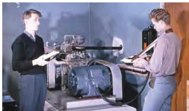
↳ Measurement with Sound Level Meter Type 2203, ca. 1970
