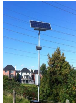
Figure 9: Noise and Vibration Monitoring Equipment
