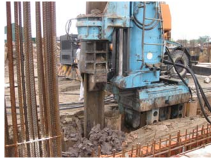
Figure 5: Silent piling using a Giken hammer
