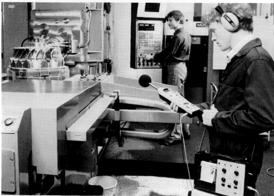
On site frequency analysis with Sound Level Meter Type 2230 and Filter Set Type 1625, recorded on Level Recorder Type 2317
