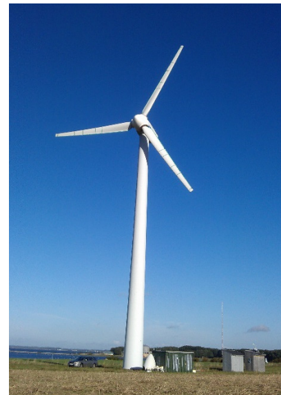
Figure 4. Vestas V27 wind turbine. The green strips on the blades are the tape protecting the accelerometer cables.
