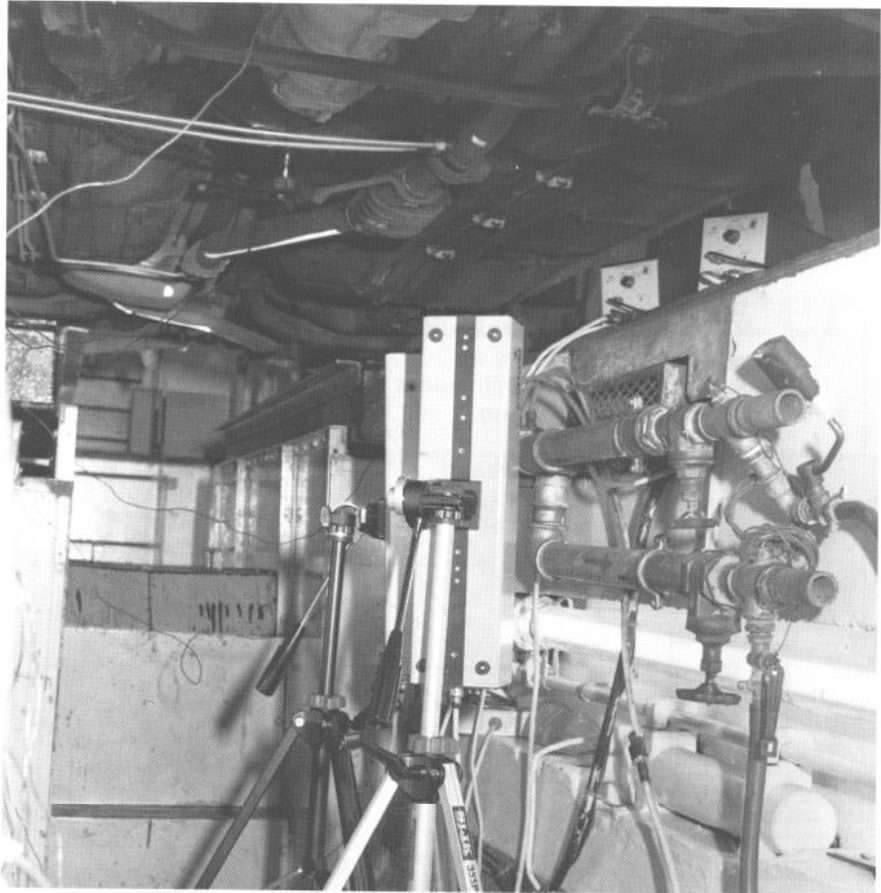
Fig.15. Making an Operational Deflection Shape Measurement on an exhaust pipe by using two lasers (photograph courtesy of The Ford Motor Company (UK) Ltd)
