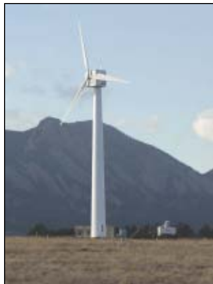
Fig. 4 A three-blade 100 kW turbine generator at NREL's facility. This configuration runs into wind and tends to be quieter than designs using two blades
