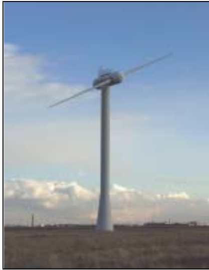
Fig. 3 This 600 kW wind turbine at NREL's facility is used to investigate the noise produced by typical downwind two-blade designs
