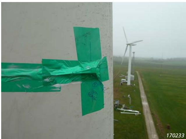
Fig. 5. Accelerometer and cable fitted to the blade (helicopter tape visible)
